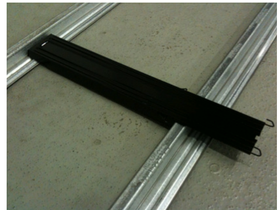
Figure 4 – Installing the Link Channel
