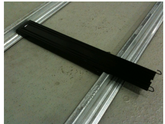
Figure 4 – Installing the Link Channel
